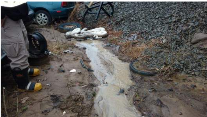
Concentrated runoff from vehicle storage area entering a drainage structure. Filter sock placed by City.
