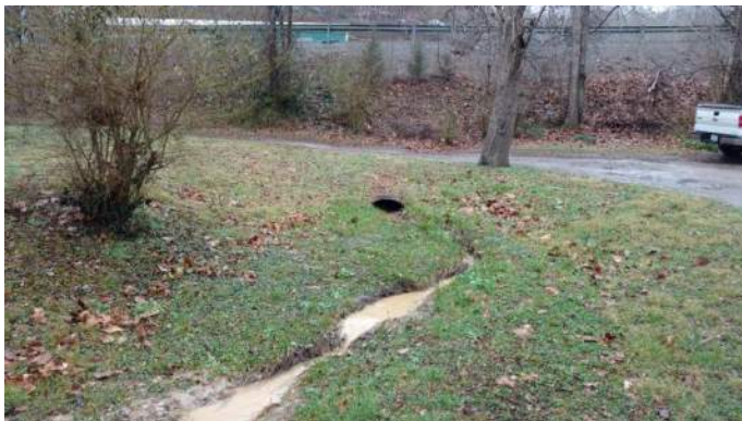
Downstream end of culvert under Louisville highway, discharging to tributary.
